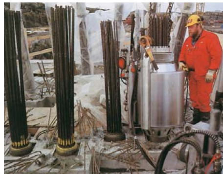
Fig. 20: TENSAM 9750 kN stressing jack stressing 37 x 0.6" anchors
